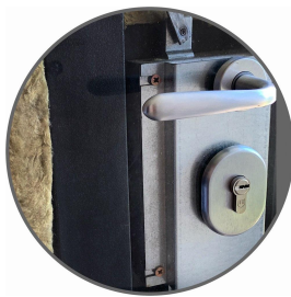
Lock protective box
